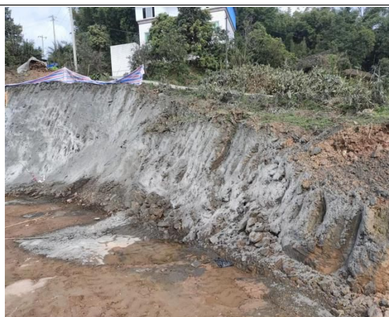
左岸厂房边坡喷护
