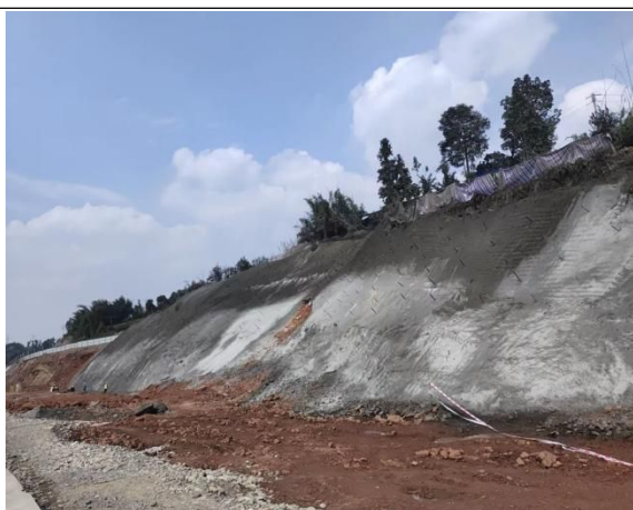
左岸厂房边坡喷护
